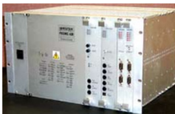
Figure 7. Prismic A30 excitation controller
