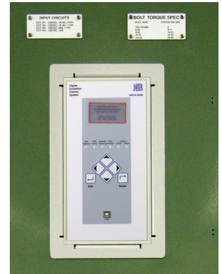
Figure 8. DECS-250N with escutcheon plate mounted in panel.
