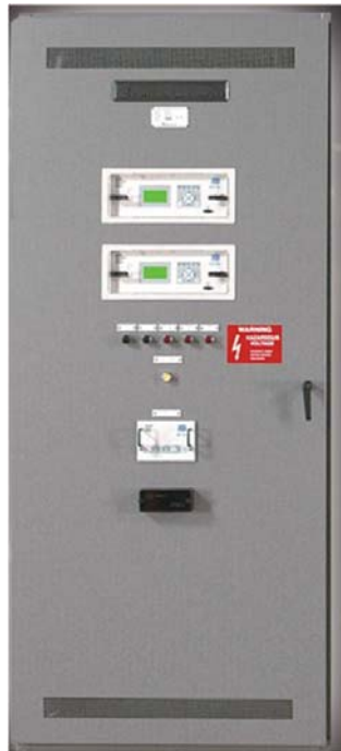
Figure 37: Dual Controllers are the Preferred Method for Backup
